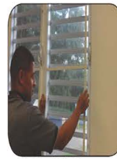
Install or repair window & door screens.
