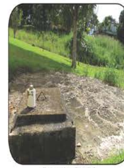
Keep septic tanks sealed.
