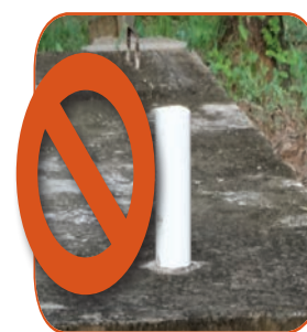
Cover ventilation pipes
