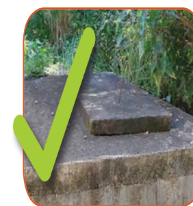
Septic tank with concrete cover
