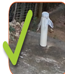
Septic tank ventilation pipe with screen mesh
