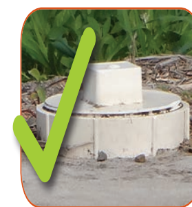
Septic tank sealed with PVC cap
