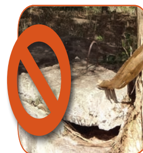
Repair broken septic tank covers
