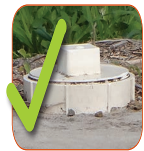
Septic tank sealed with PVC cap
