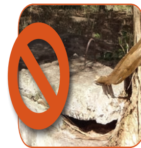
Repair broken septic tank covers
