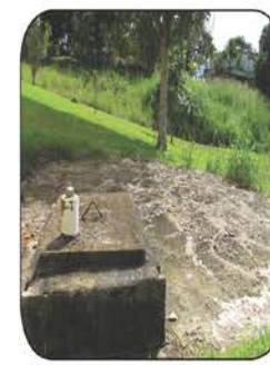
Keep septic tanks sealed.
