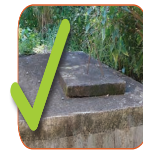
Septic tank with concrete cover
