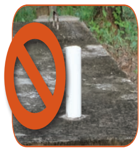
Cover ventilation pipes
