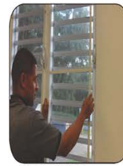
Install or repair window & door screens.
