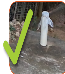
Septic tank ventilation pipe with screen mesh
